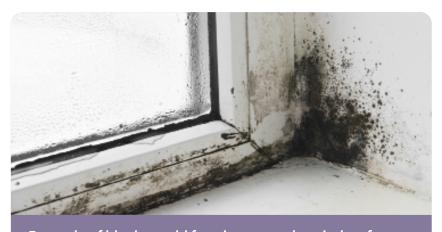
Example of black mould forming around a window frame
